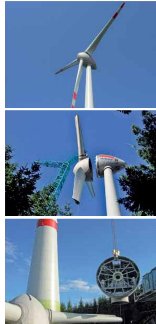
Installation of ENERCON E-126/7.5 MW at Ellern wind farm. Teams install turbines in record time.
